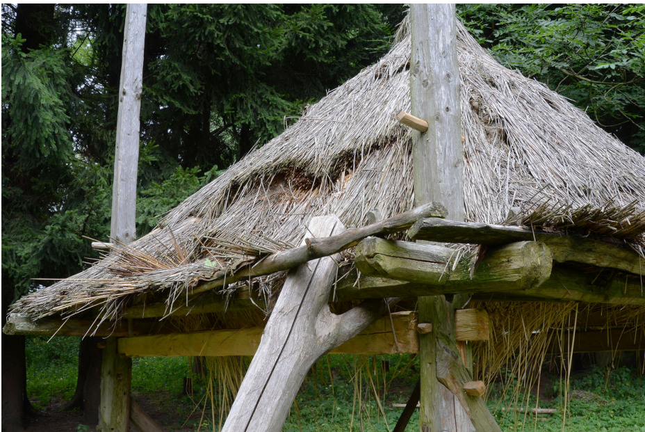
Hay barrack, roof cosntruction in detail.
